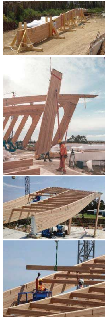
Figure 11: MACA construction process
