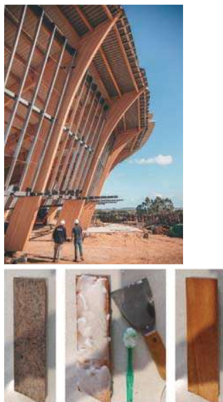
Figure 12. Steel structure for supporting the envelope and experimental tests with oxalic acid to remove the stains [23].
